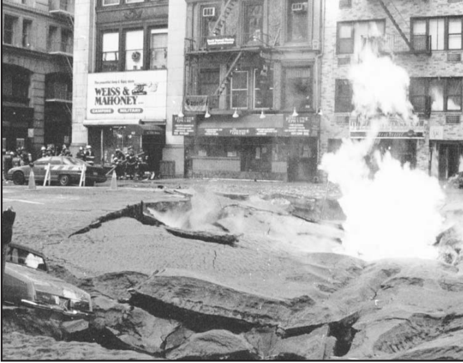
Water main break on Fifth Avenue and 20th Street in Manhattan on January 2, 1998, undermined the roadway, causing the street to collapse. The collapse, in turn, undermined the gas main and electric cables, resulting in a substantial gas fire that took two hours to control.
