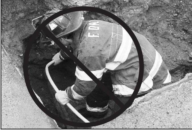
This is an example of what not to do! Never attempt to shut the flow of gas from a ruptured plastic gas line due to possible static electricity charge on the pipe. Please note that this is a training photo; not one taken at an actual incident.
